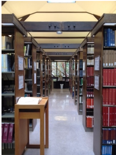
BEFORE: Asbestos floor tile
